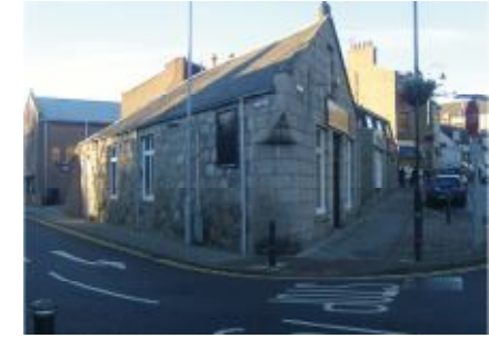
Note how this building on the corner compensates for the awkward angle and slope of the site.
